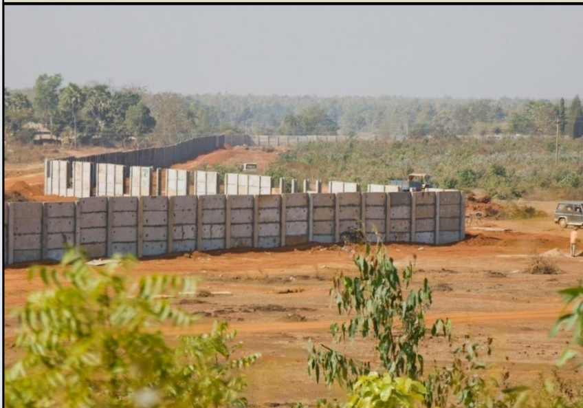
Completed boundary wall
