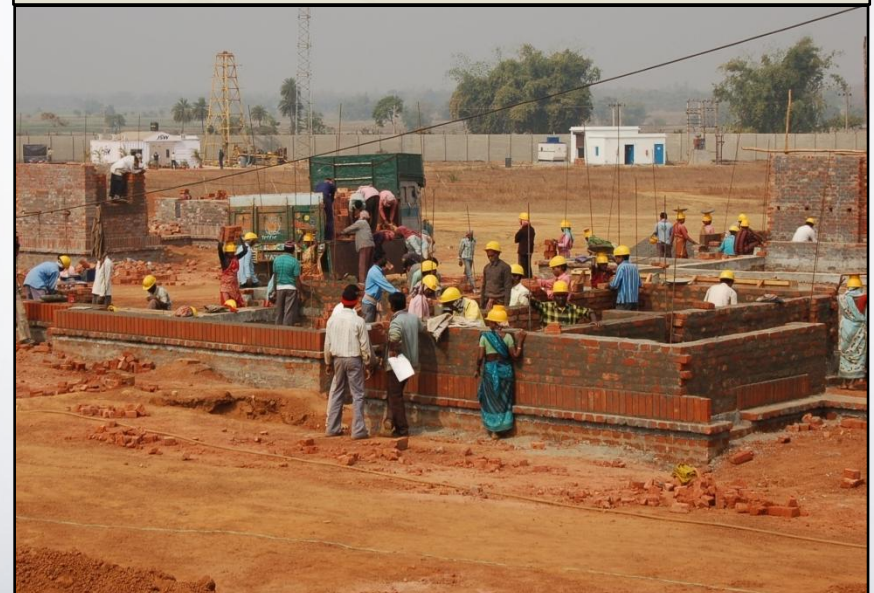
Township work in progress
